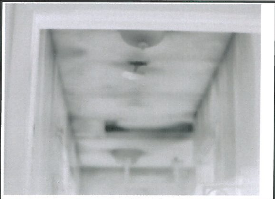
Hallway ceiling at second floor
